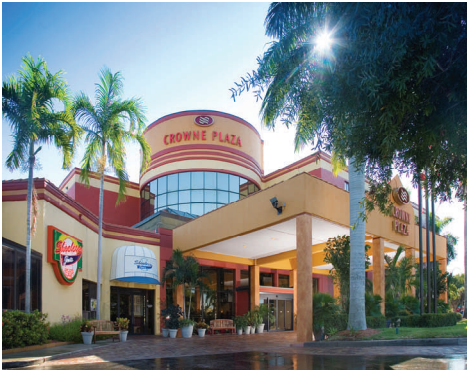
Crowne Plaza Fort Myers at Bell Tower Shops
